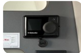
Regulator for the heating
